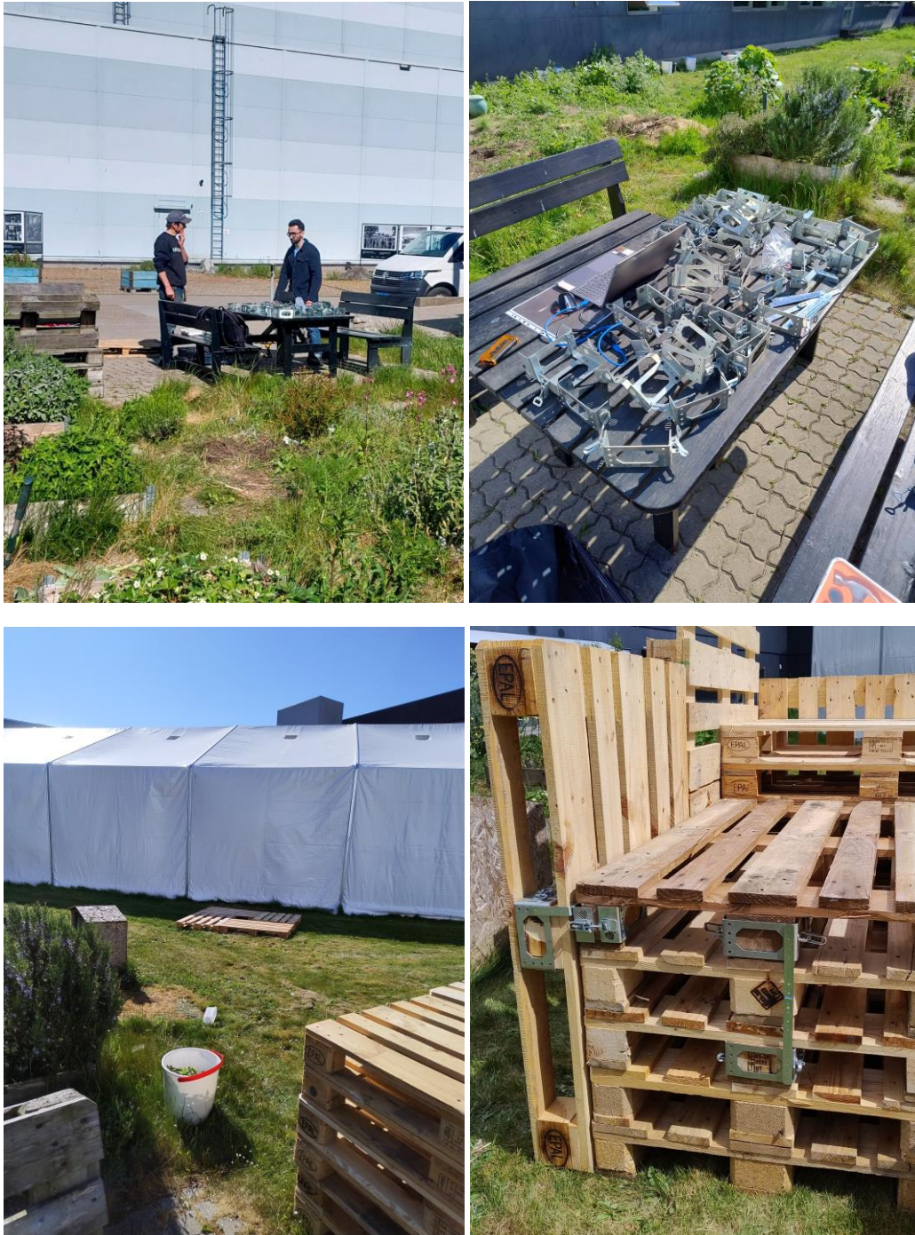
Figure 26. Look and Feel prototype under construction.
